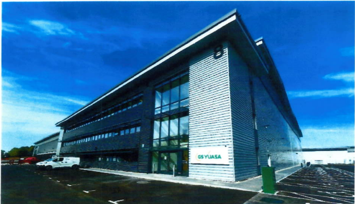
GS Yuasa Battery Europe Ltd head office & GS Yuasa Battery Sales UK Ltd
