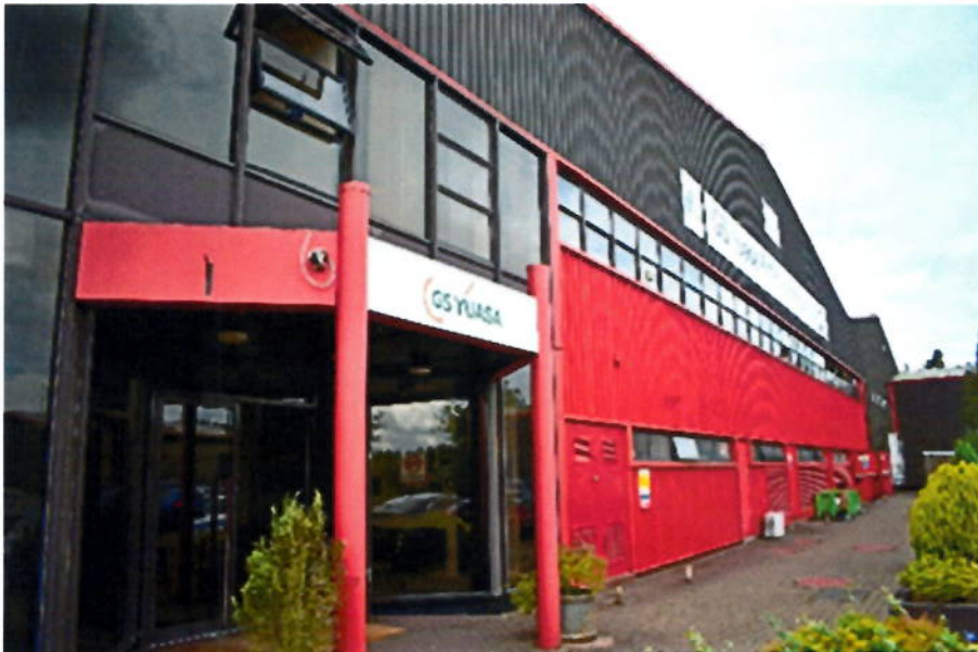
GS Yuasa Battery Manufacturing UK Ltd
