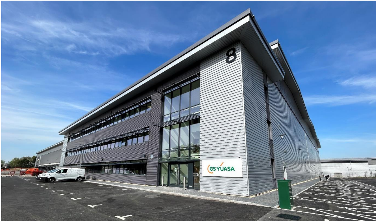
GS Yuasa Battery Europe Ltd HQ & GS Yuasa Battery Sales UK Ltd
